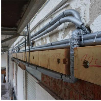
Figure 4.a) Installation of the water and sewage distribution pipes (Gumpp & Maier GmbH)
