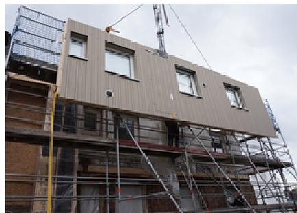
Figure 8.b) Erection of the prefabricated wall elements
