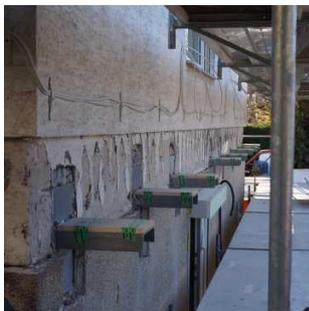
Figure 8.a) Steel supports of the timber frame wall
