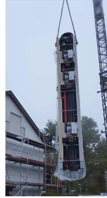
Figure 4.b) Cranage of the shaft on site (Gumpp & Maier GmbH)
