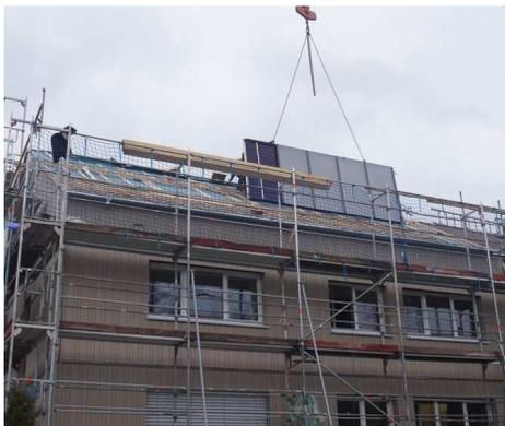
Figure 5.a) Installation of the solar thermal collector (Gumpp & Maier GmbH)
