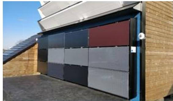
**Figure 2:** The outdoor colored and textured PV façade demonstrator installed at SolarBEAT, Eindhoven.
