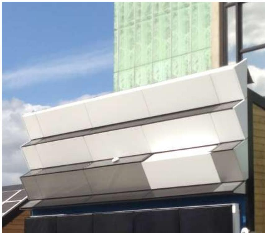
Figure 4. Close-up of full-scale ZigZagSolar demonstrator at SolarBEAT test site, Eindhoven, The Netherlands.
