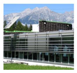
**Daylight solution:** exterior louvers with varying distance between slats optimized for location, additional screen for luminance control
